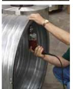
4. With the Ductmate Inner Ring firmly pressed against the edge of the ductwork, start attaching the ring to the inner liner starting at the split and working in one direction. Make sure the ring is properly seated as you attach it to the liner.
