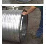
3. Slide the Ductmate Inner Ring over the inner wall of the ductwork. Seat the ring firmly against the edge of the Spiralmate flange.
