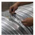
11. Slide the closure ring over the mating flanges and insert the bolt.
