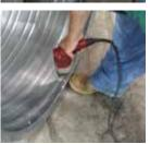
5. The Ductmate Inner Ring should be attached using rivets, screws, stitch welds or tack welds every 12" to 18" on center. The Inner Ring was designed to incorporate a minor gap at the split. This gap will not affect the performance of the finished system. An overlap is not recommended as it may hinder the installation of the Closure ring.
