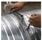
12. Tighten the bolt on the closure ring until it makes even contact around the circumference of the duct sections. Tap around the joint with a hammer if necessary to seat the flange while tightening the bolt.
