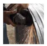
7. Welds may need to be ground down before proceeding with the application of the Neoprene gasket. No fasteners with a head larger than 1/16" in height may be incorporated when attaching the Ductmate Inner Ring to the Spiralmate flange.
