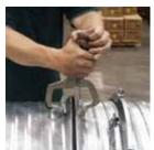
10. Finish the connection by slipping the outer closure ring over the end of the duct. Align the flanges using the Spiralmate alignment grips.
