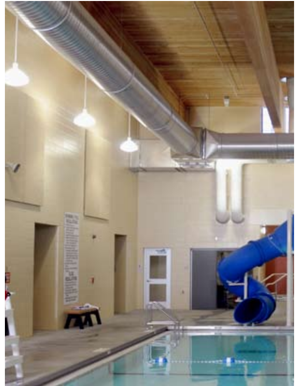
Spiralmate is available in specialty metals that withstand corrosive environments like this indoor swimming pool.
