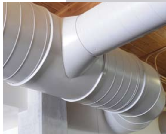
Detail: Spiralmate connections eliminate costly sealing, and are virtually invisible at a distance.
