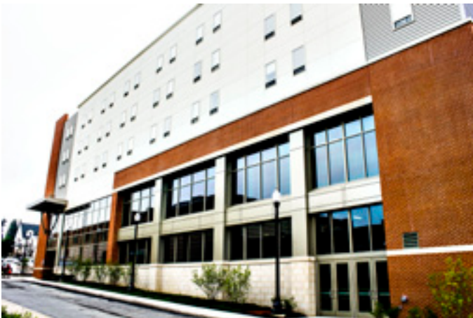
Indiana University is spending $15 million to build a student housing and recreation center on its Indiana, Pa., campus.
